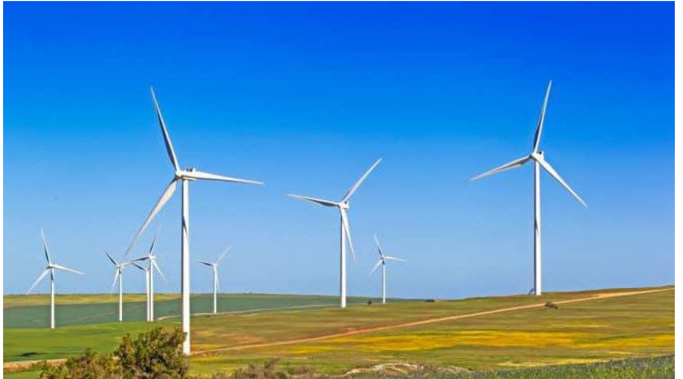
Wind turbines producing electricity.
